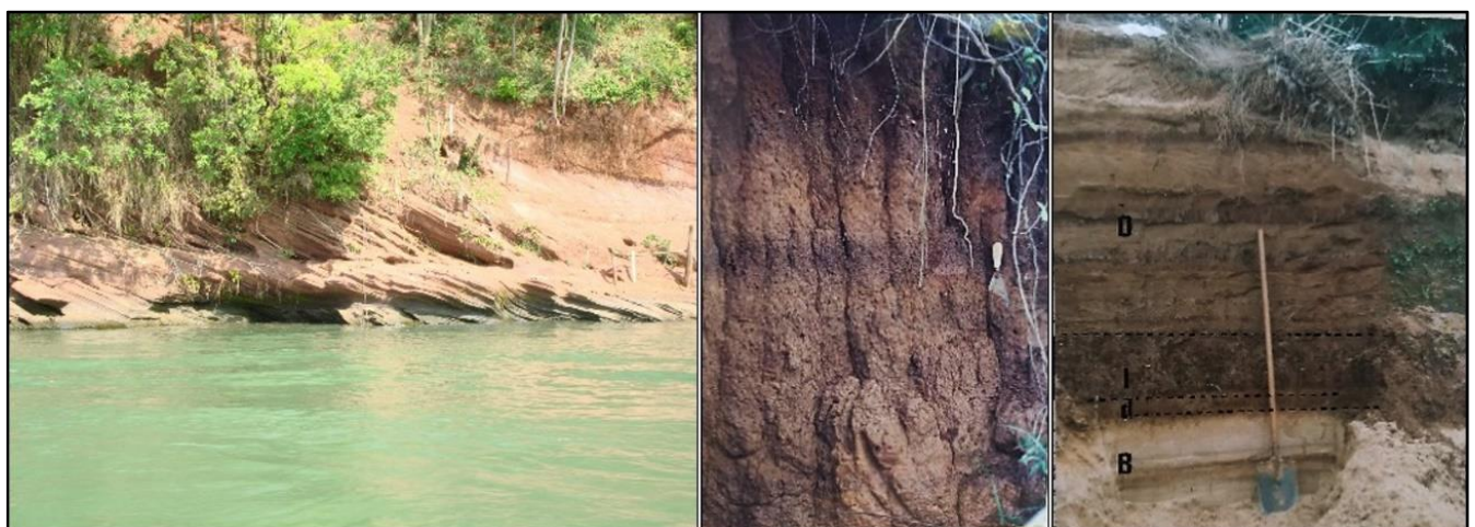
Figure 4. Banks of the Upper Paraná River in the study reach: (L) left vertical bank formed by the sandstone of the Caiuá Fm.;
