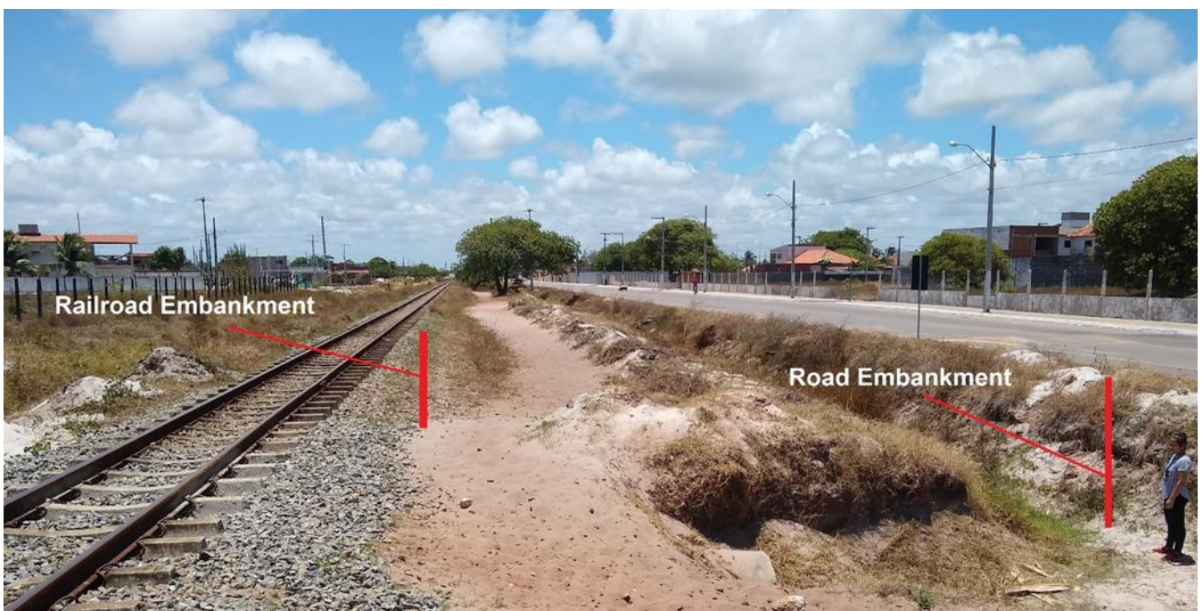
Figure 5. Landfills for railroad and highway – Cabedelo. It is possible to visualize the unconsolidated sediments of the Quaternary between the two landfills. Photo: Authors (2020).
