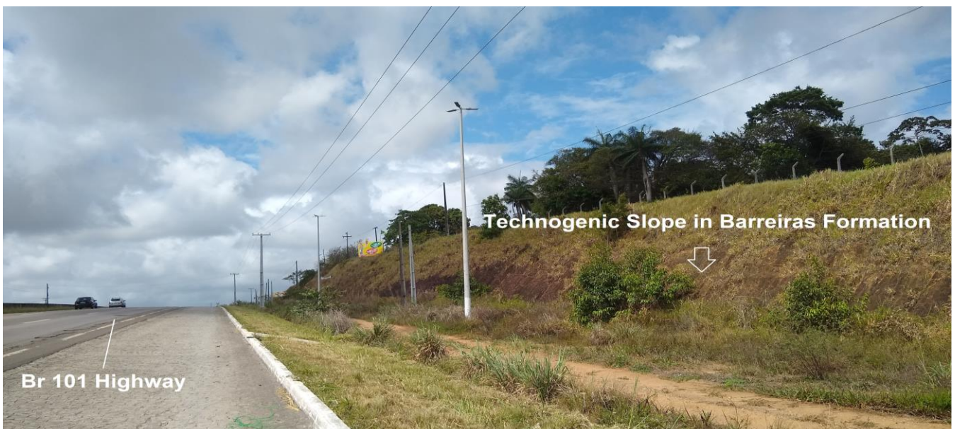
Figure 12. Cut in the Barreiras Formation. BR 101 Highway. Municipality of Conde. Photo: Authors (2020).
