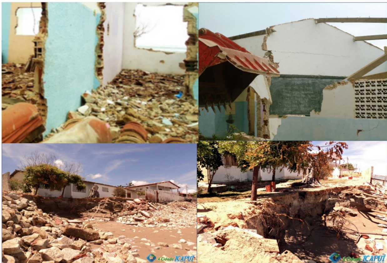
Figure 20. Damage caused by coastal erosion to accommodations at Praia da Barrinha between 2002 and 2010. Source: Blog "A Cidade Icapuí."
