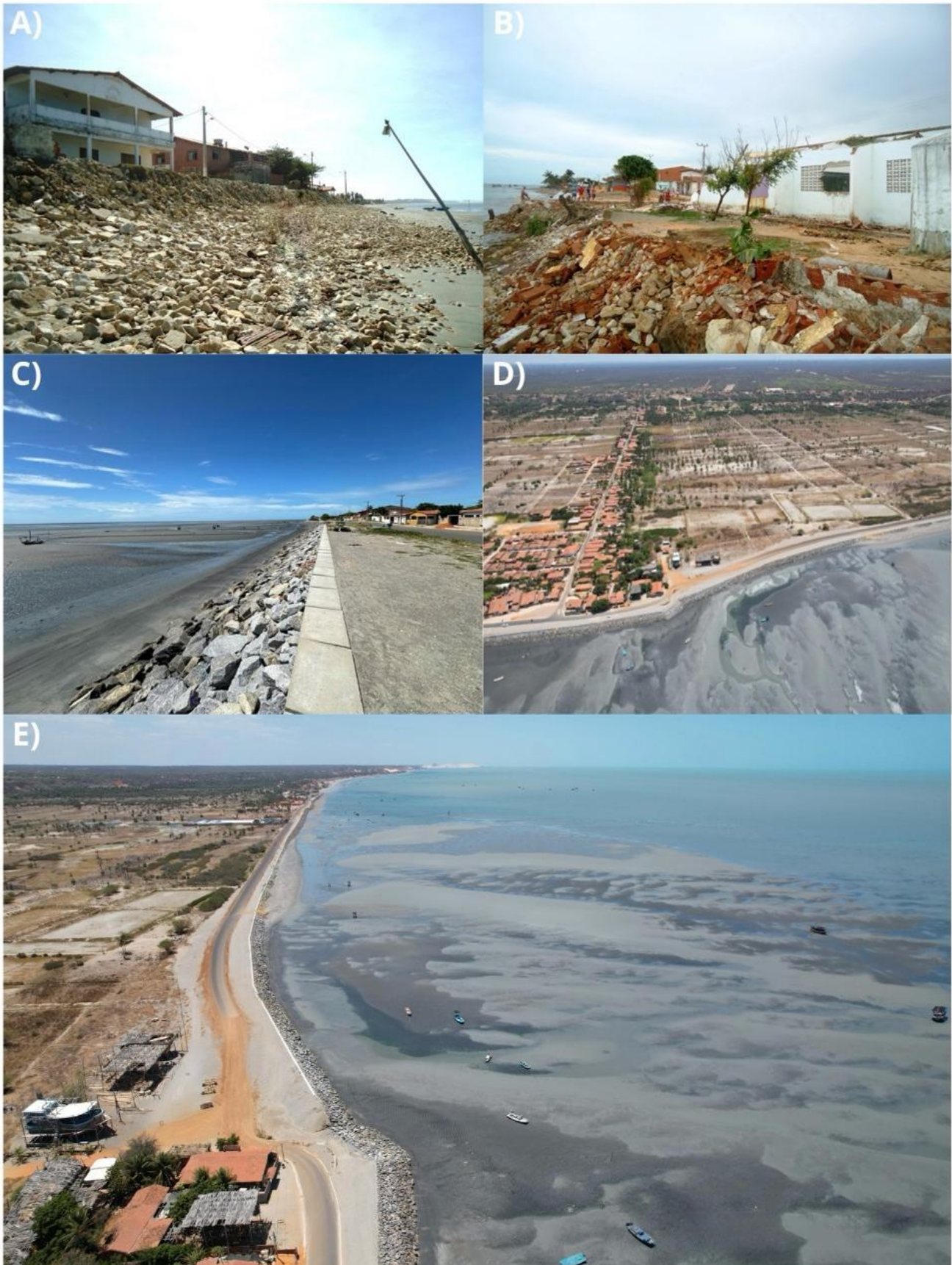
Figure 22. Evolution of a stretch of analyzed shoreline in sector 3. A and B) Photographic records from the period of intense erosive processes and the consequent damage to the structures built in the area in 2010; C, D, and E) Photographic records from 2024 obtained in the same stretch.
