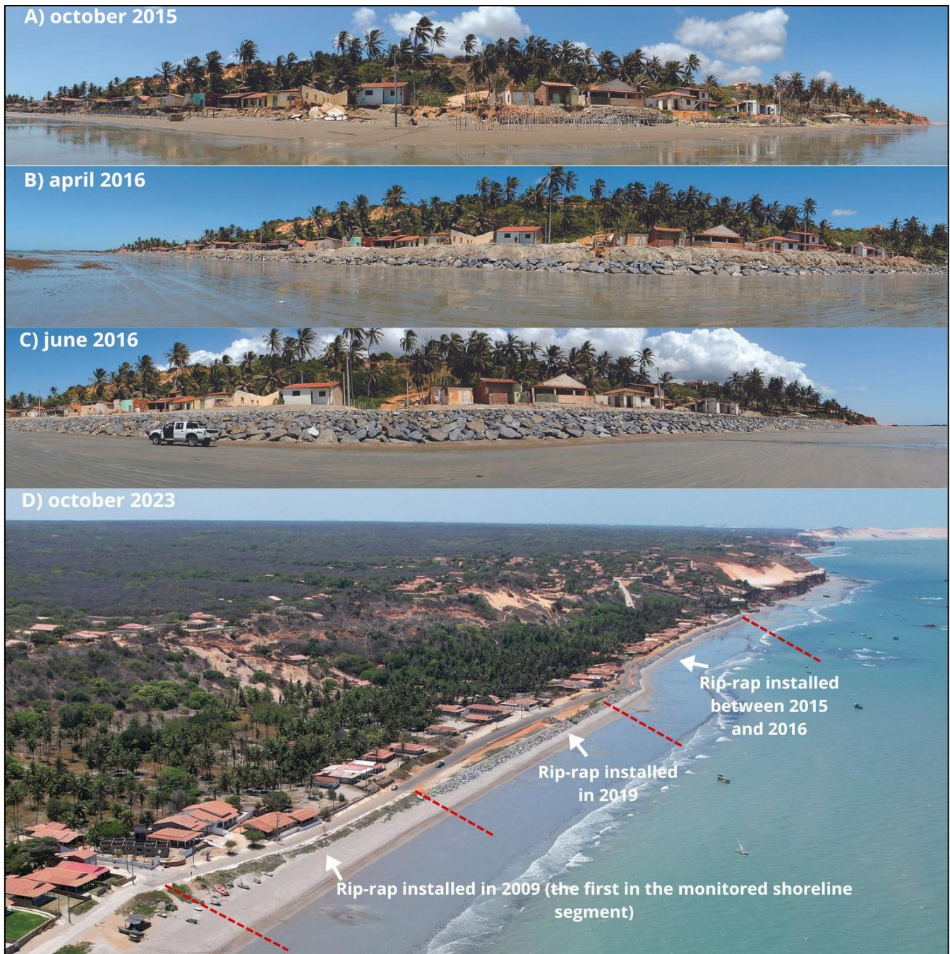
Figure 18. Evolution of the process of installing a rock revetment at Barreiras de Baixo Beach between 2015 and 2023. A) Section of Barreiras de Baixo Beach with the accommodations destroyed due to erosive processes and the retreat of the shoreline. The presence of temporary structures for tidal and erosion control is highlighted; B) Beginning of the installation process of the rock revetment to prevent shoreline retreat; C) Completed installation of the rock revetment; and D) General overview of the rigid structures built in the analyzed sector between 2009 and 2019.
