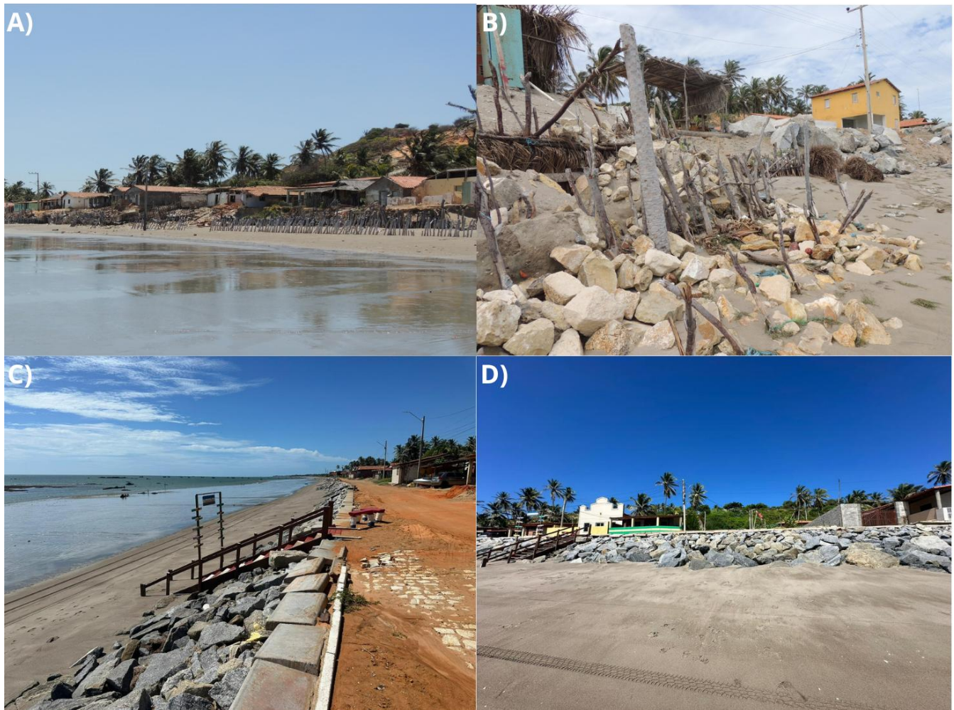
Figure 17. Containment measures are used to prevent the retreat of the coastline and mitigate the action of the tides. A and B) Alignment of wooden stakes, limestone blocks, and sandbags – 2015; C and D) Use of rigid structure in the form of Rip-rap in the same location to prevent the retreat of the coastline – 2024.
